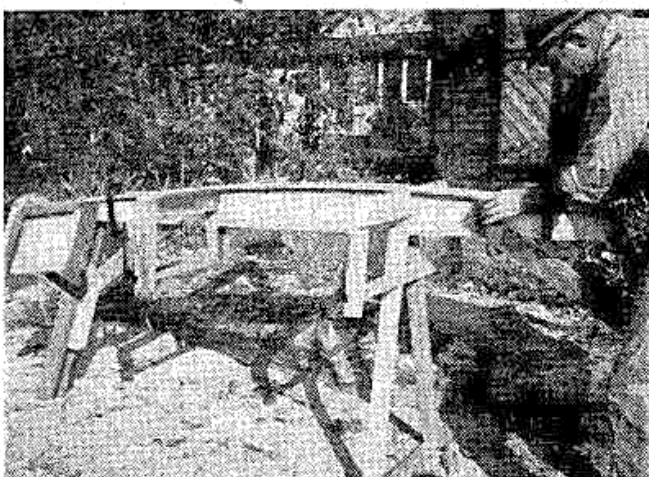
Mould frames, form set up. Transom, keel, stem attached.
