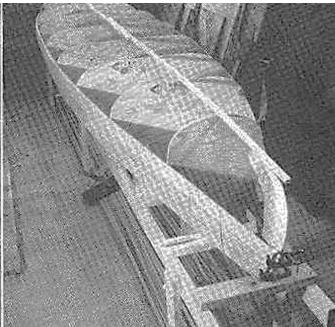
Redwood strips are tacked to the templates, and edge-glued. Drive brads through into the templates before putting on fiberglass cloth.
