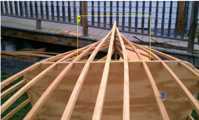
Image Notes 1. This deep V is unnecessary and undesirable. I figured that out too late.
